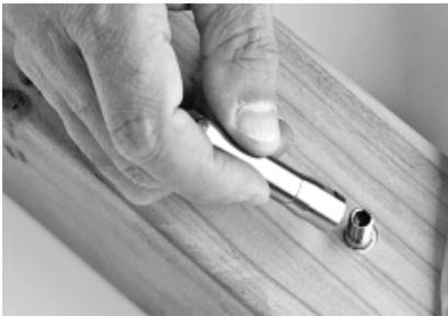
8. Make sure the post side of the Push-Lock lag is flush against the post.
